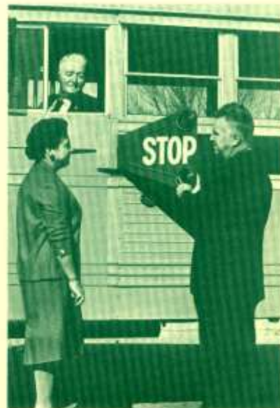
This bus stop-arm has 2 red flashing lights for better signaling. Transportation Director C. D. Stout discusses the feature with school-bus drivers Inez Long, and Ronald Henneous.
